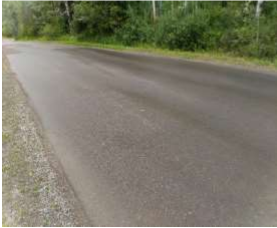
Level 3 Patch - In good condition
