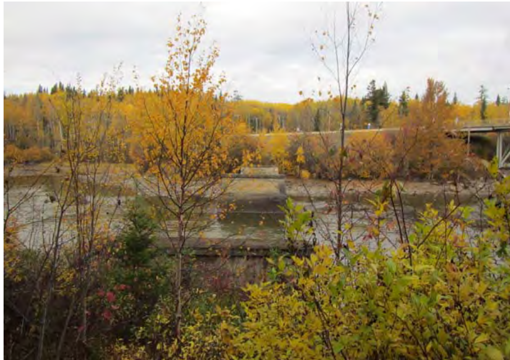
Figure 57: Old Concrete Piers across Stuart River
