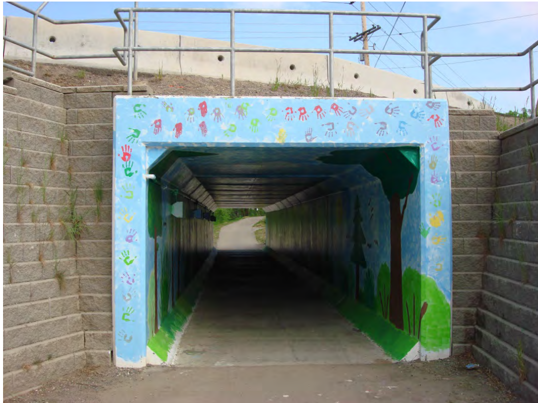
Figure 27: Heritage Trail Underpass on Highway 16, Prince George
