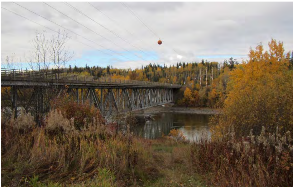
Figure 2: Stuart River Bridge
