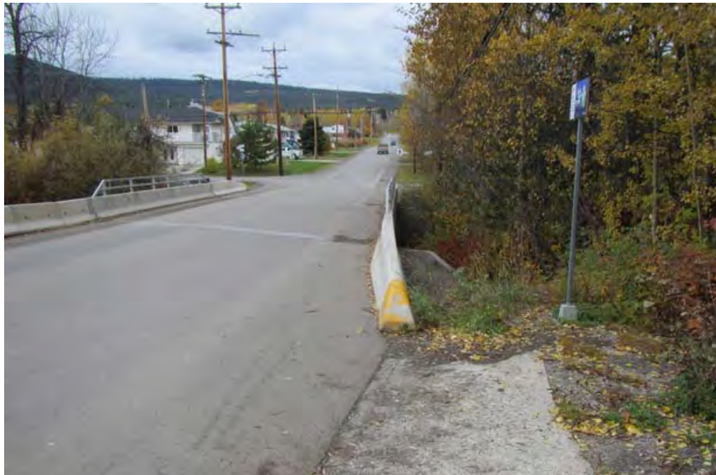
Figure 41: Douglas Avenue Bridge
