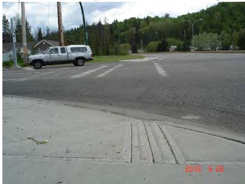
Figure 26: Sidewalk Ramp with Tactile Grooves, Prince George
