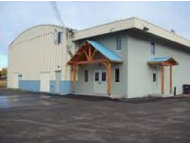
Figure 1 – Fort St. James Arena
