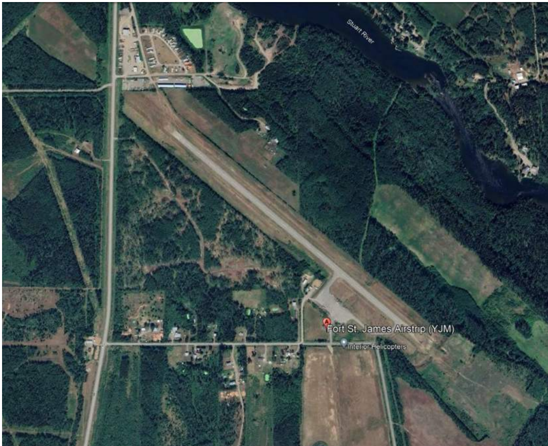
Figure 3.1.2. Fort St. James (Perison) Airport Aerial View (Existing 07/2023)
